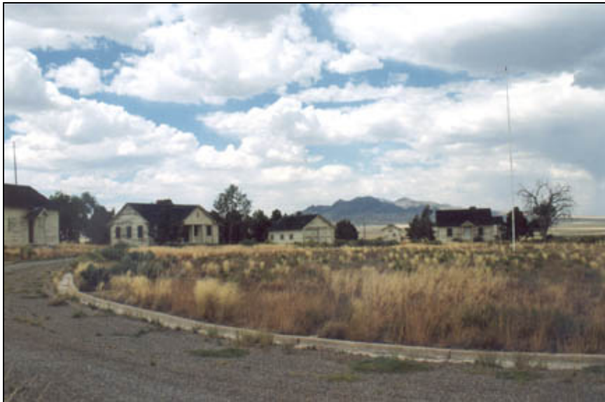
Weed-filled circular driveway ringed by deteriorating DRES buildings and empty flagpole. July 17, 2005 photograph © by Linda Moulton Howe.
