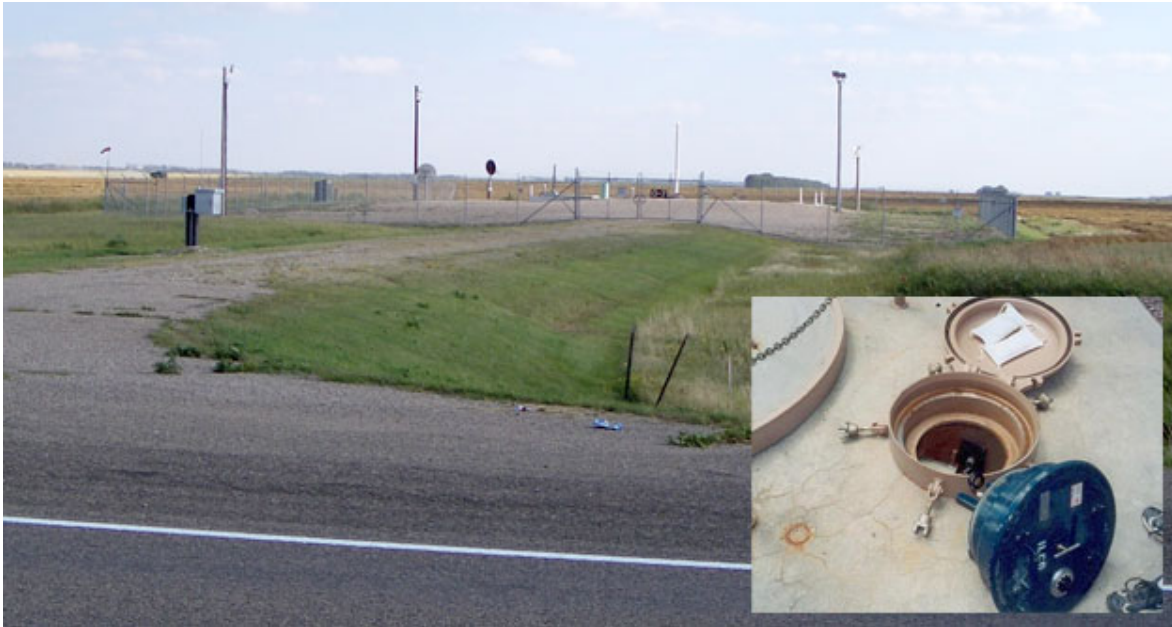
Oscar-7 Launch Facility located 24 miles north of Minot AFB, to the south of ND Highway 5W; and (inset) the personnel access hatch's weather cover flipped open with the vault door removed, providing access to the controls to open the primary door. In this instance, somebody had entered the facility triggering the outer-zone alarm, opened the weather cover, and turned the combination dial off its setting triggering the inner-zone alarm.
